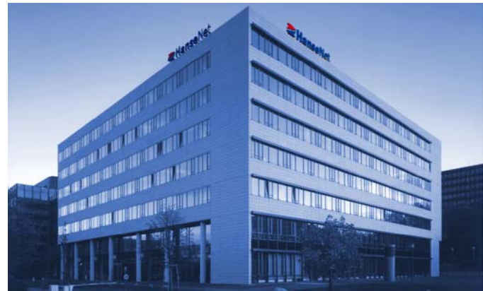
Company headquarter of HanseNet Telekommunikation GmbH, City Nord, Hamburg © Palladium Photodesign, Köln, Germany / Photo: Oliver Schuh
